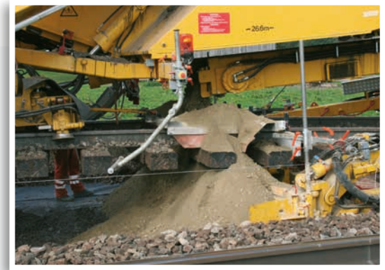
Installation of new FPL material
